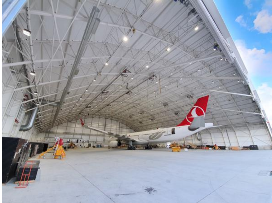
Ascent Aviation hangar at another operations center - Roswell hangar will be similar once it is completed. Photo courtesy of Ascent Aviation.
