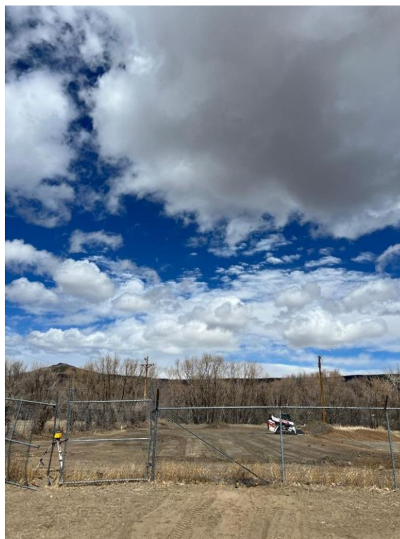
Ramel Family Farms greenhouse grading
