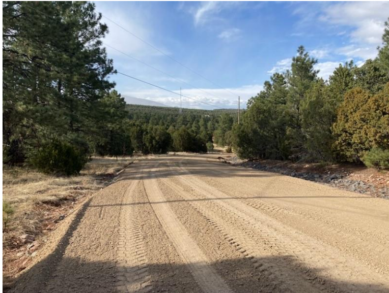
Newly renovated entry road provides year-round access to the park.
