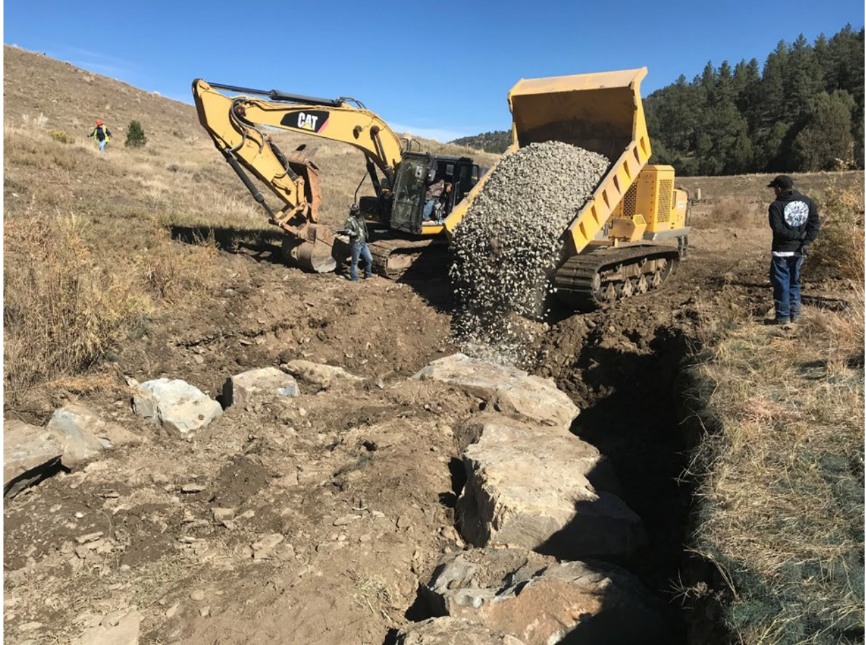
Construction of a cross vane in the stream channel, October 2020
